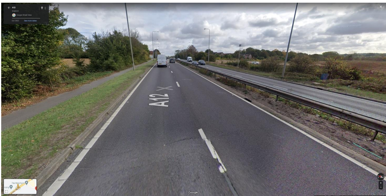
Plate 3.1 – Existing D2AP A12 south of Rivenhall End looking north
