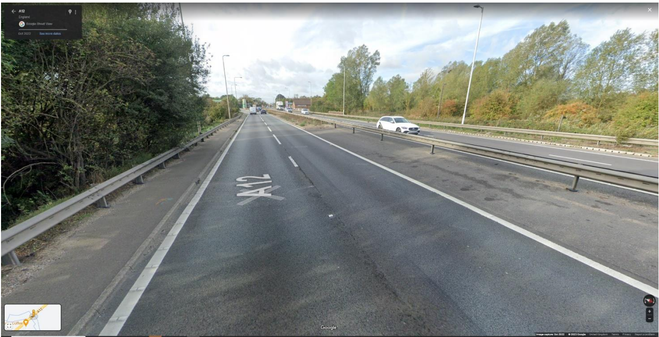
Plate 3.2 – Existing D2AP A12 north of Rivenhall End looking south
